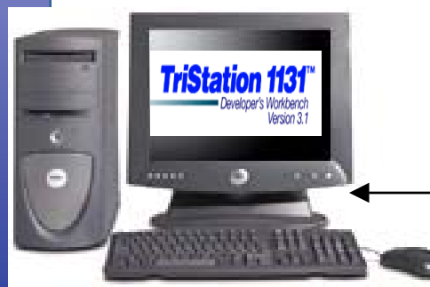
Eng/Operator Station Running Tristation
